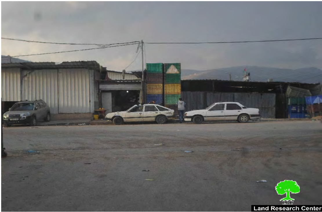
Beita-Nablus: Vegetables central market before demolition. February 2016
