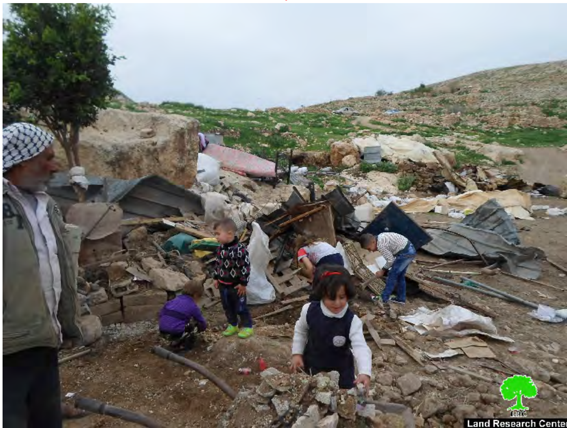
Hebron village of Beit Al-Rush: Israel Army and Civil Administration while demolishing structures on January 2016
