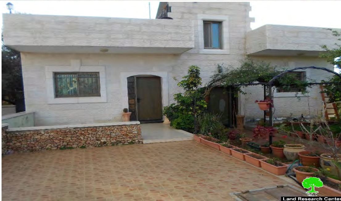
A threatened house in Badras village
