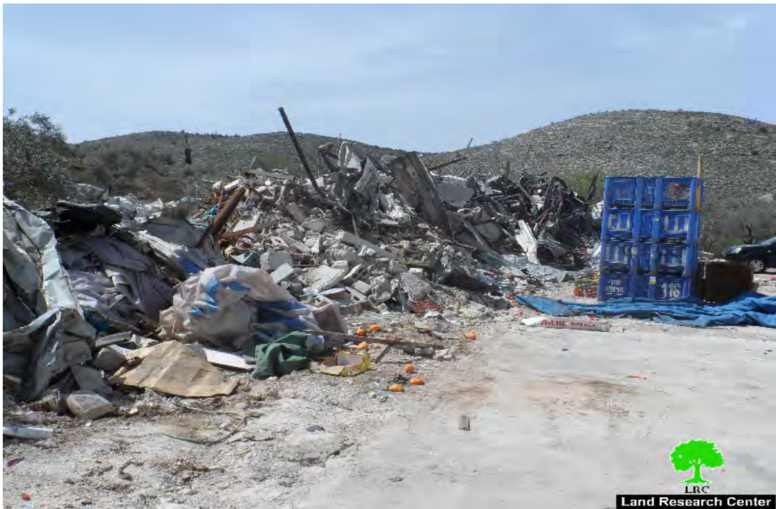
Beita-Nablus: Vegetables central market after demolition. March 2016
