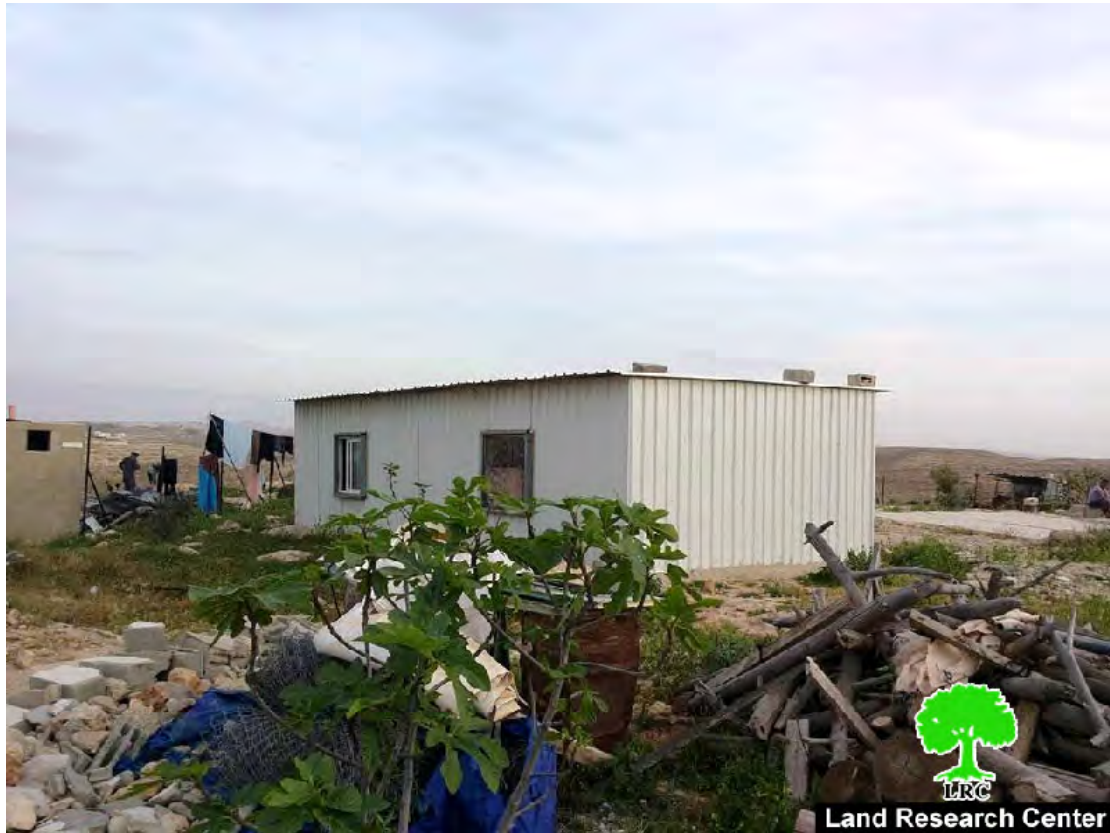
Um Al-Kheir- Masafer Yatta: stop-work orders on a Al-Hadhaleen family residence on March 2016
