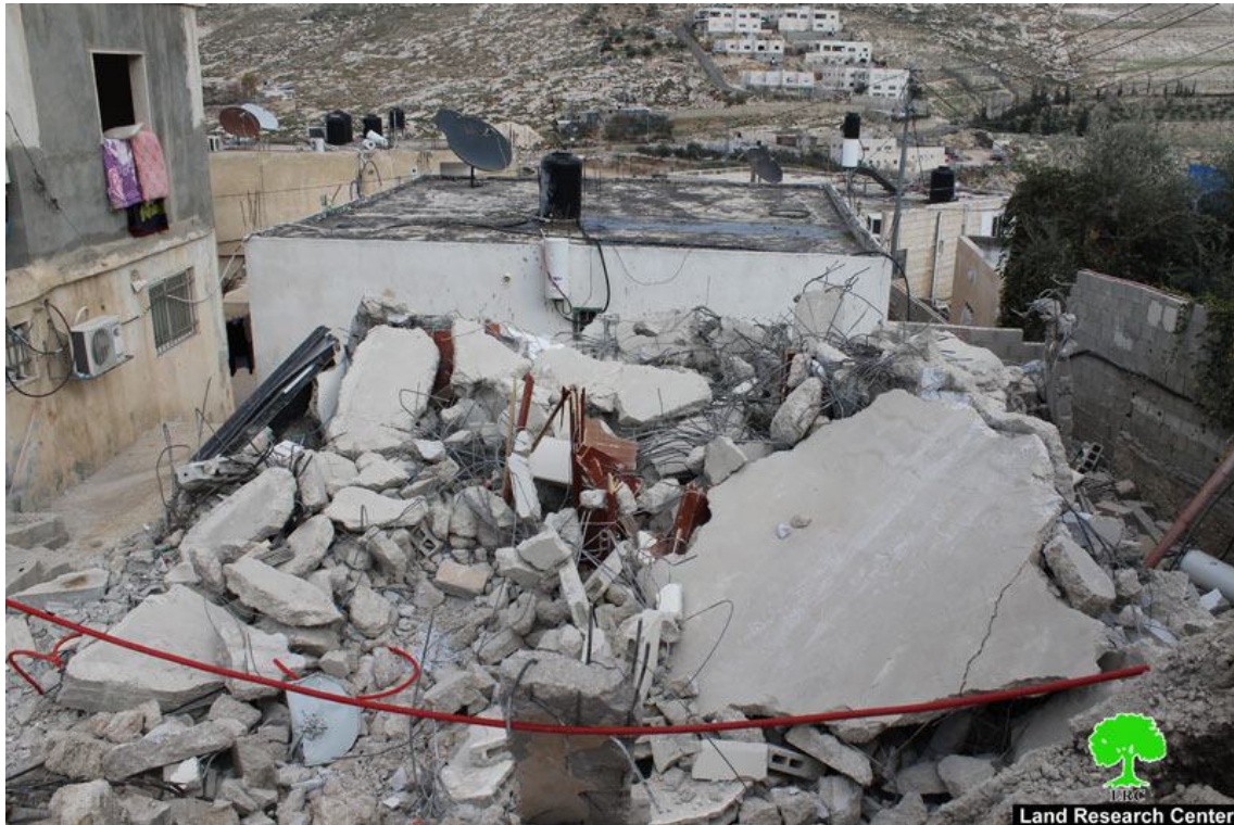
Bashir's house that turned into wreckage
