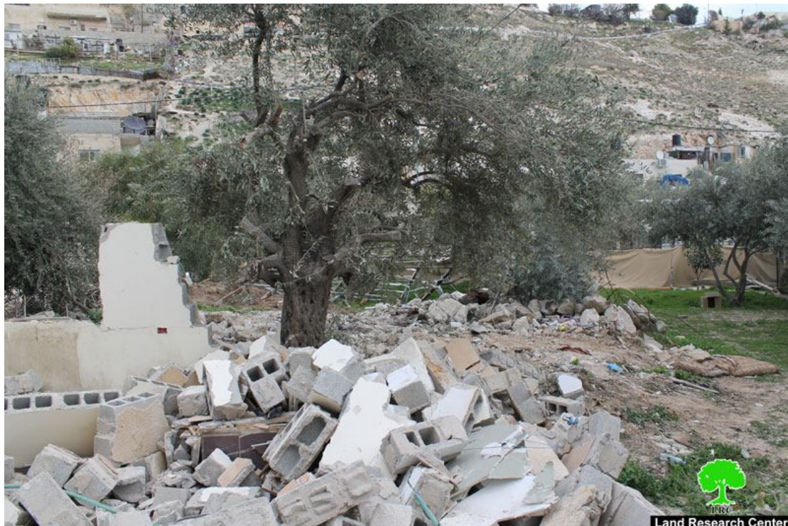
Mashahra's residence destroyed
