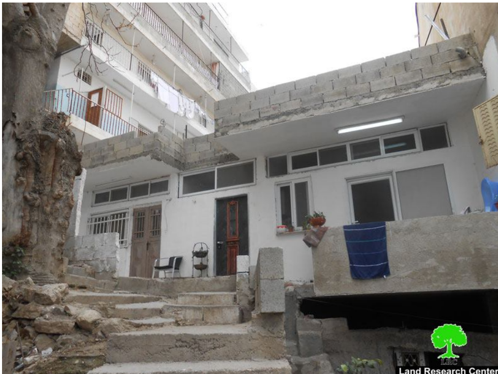
Saim's threatened structure
