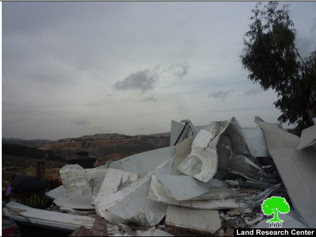
The damage ensued by the bulldozers after demolition
