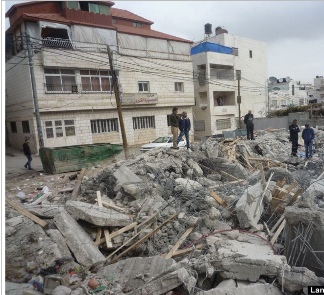
A picture of the building reduced to rubble in Al Eisawaya
