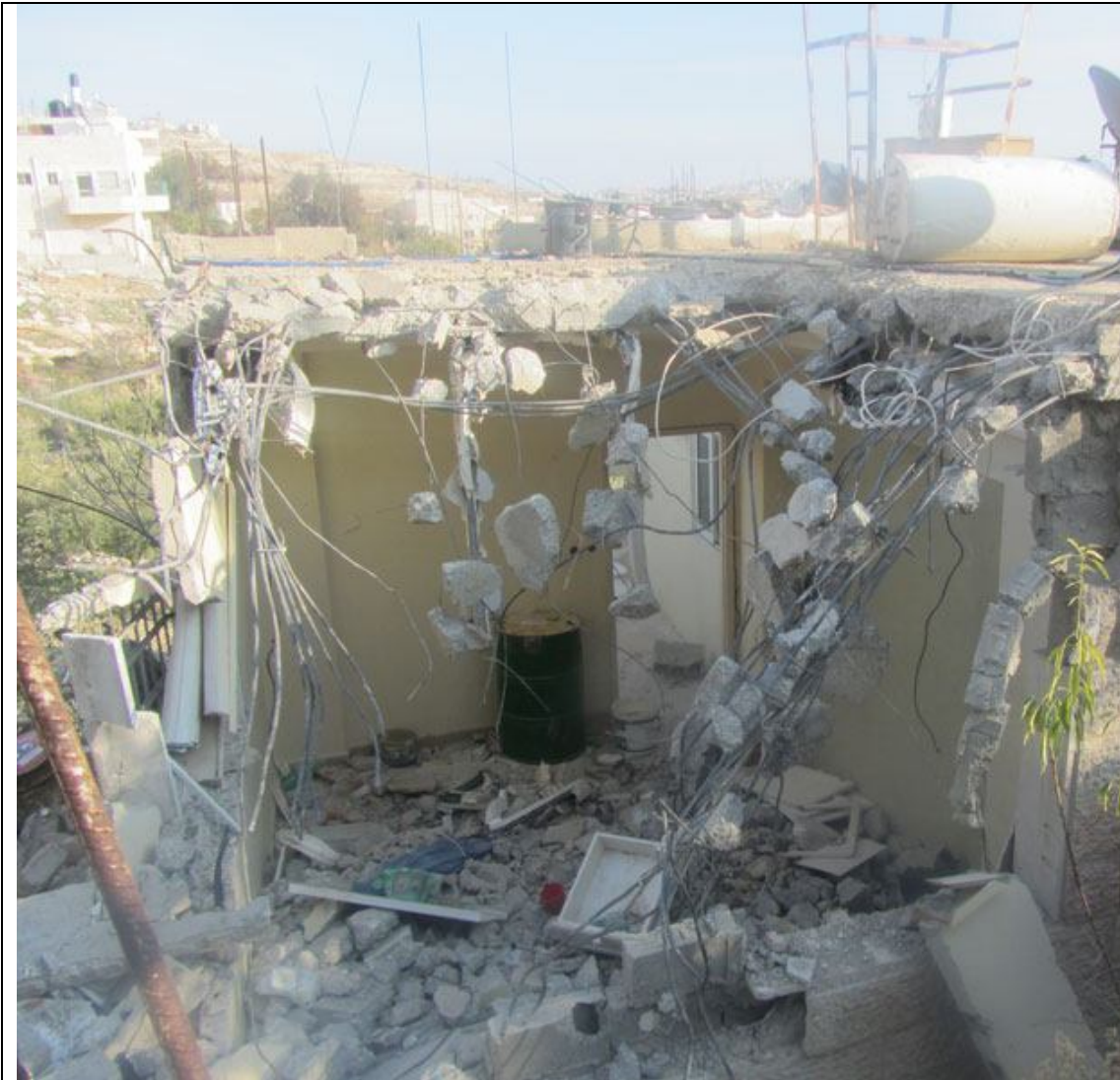
Abu Ter's house after being demolished
