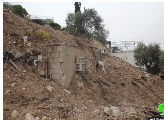
Ayman's residence 7 feet under
